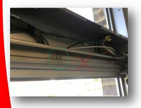
DO NOT lift track ABOVE factory settings as the door will not be level. Keep the track free of debris and never put additional screws or fasteners in it as they may hit the roller bearings and stop the window from self closing.
