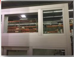
DO NOT expose top of window during construction by leaving the cavity open for the air curtain. Rain and snow may damage the electrical components.
