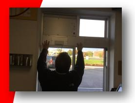
DO NOT overtighten the header cover.
